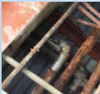
***Top: protecting the church windows from impending construction; Above left: demolition of Priory garage; Above right: corroded and rusted plumbing in Priory building.***
